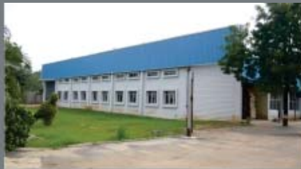
Hydraulic Valves Plant
